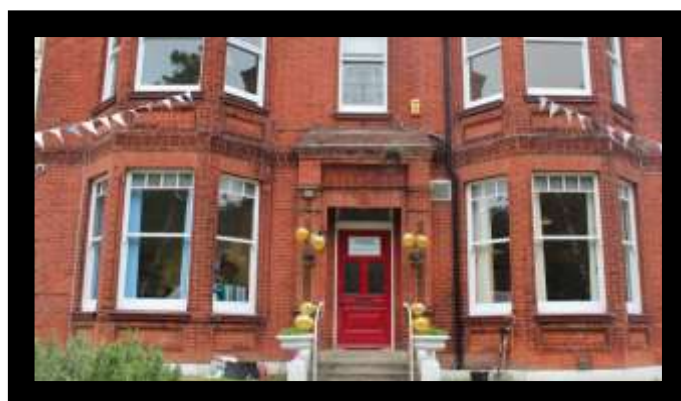
Host Site: Preston Park Recovery Centre
